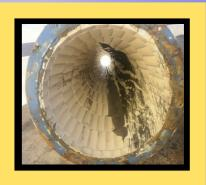
Tiles are removed and the substrate repaired and then blasted.
